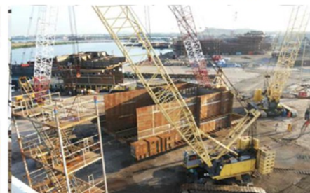
LIFTING UPPERHULL BLOCK
