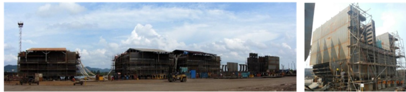
Fabrication of Pontoon & Columns MODU Intervention Semi-submersible Vessel
