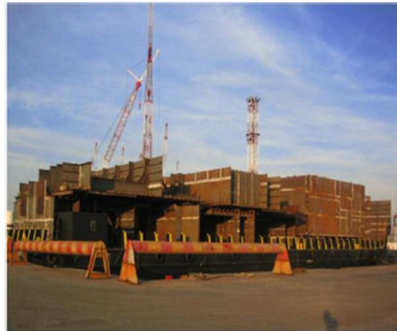
PROJECT HELIX UPPERHULL BLOCKS - LOADED ON BARGE DELIVERY BATAM TO JURONG SHIPYARD
