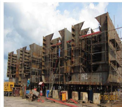
PROJECT HELIX - PONTOON BLOCKS
